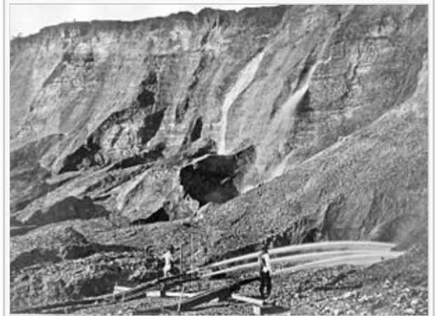
Gold miners excavate an eroded bluff with jets of water [edit] at a placer mine in **Dutch Flat, California** sometime between 1857 and 1870.
